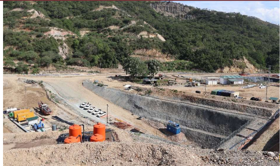
Portal & Underground Tunnel (decline) Construction
