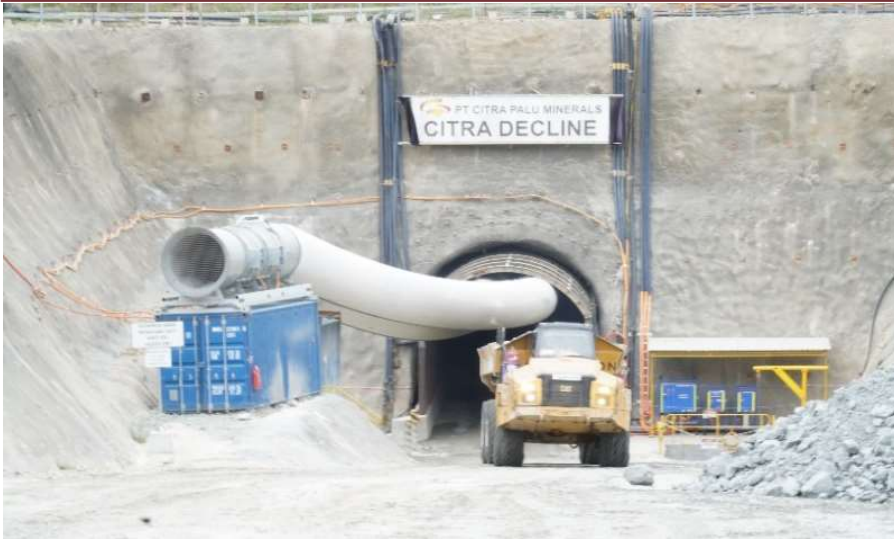
Portal & Underground Tunnel (decline) Construction
